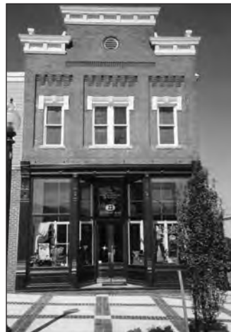
In the 1990s, Peerless stepped in to save Wire Hardware, one of the few examples of 19th-century commercial architecture in Rockville.
