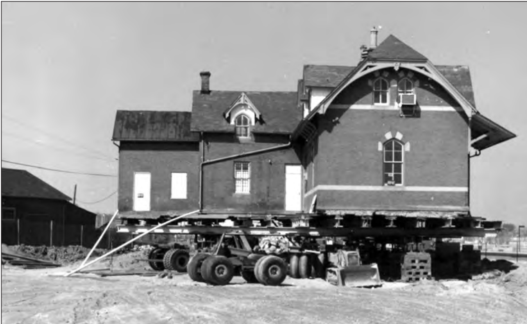
Rockville's B&O Railroad Station on the move, 1981. Faced with the possible demolition of this 1873 treasure, Peerless and the City of Rockville successfully advocated for relocating it out of the way of the Metro line. Photograph by John Spano.
